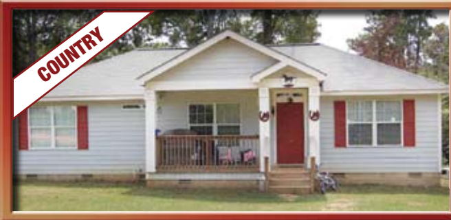
HOME IS LIKE NEW. Open concept 3/2 in the country. Very clean & well kept. House sits on over 1 acre. Perfect starter home or for small family. Close to town. REB# 67182141. $119,000
