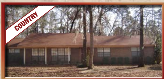
BEAUTIFUL home completely remodeled with new paint, crown molding, recessed lighting, French doors! On corner lots with shade trees plus bus stops in front of home. REB# 53898948. $159,500
